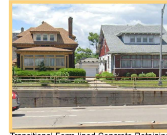
Transitional Form-lined Concrete Retaining Wall to Residential/Greenery
