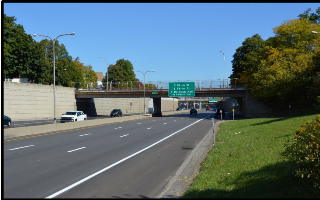
View looking north from the eastbound direction of the Kensington Expressway toward the proposed south tunnel portal.
