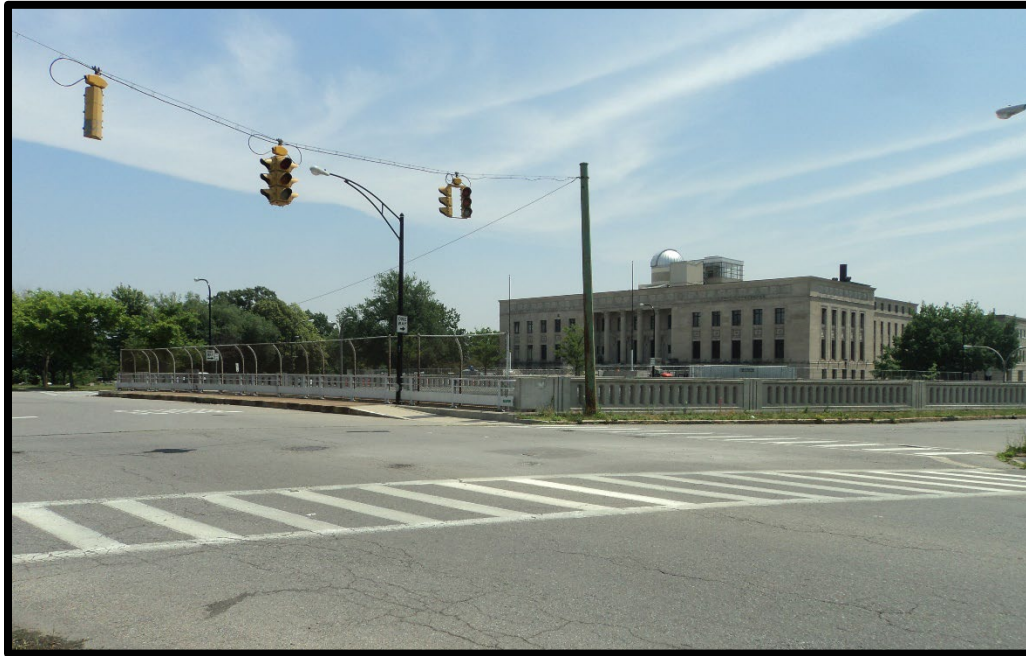
View looking southeast from the corner of Northampton Street and Humboldt Parkway southbound.
