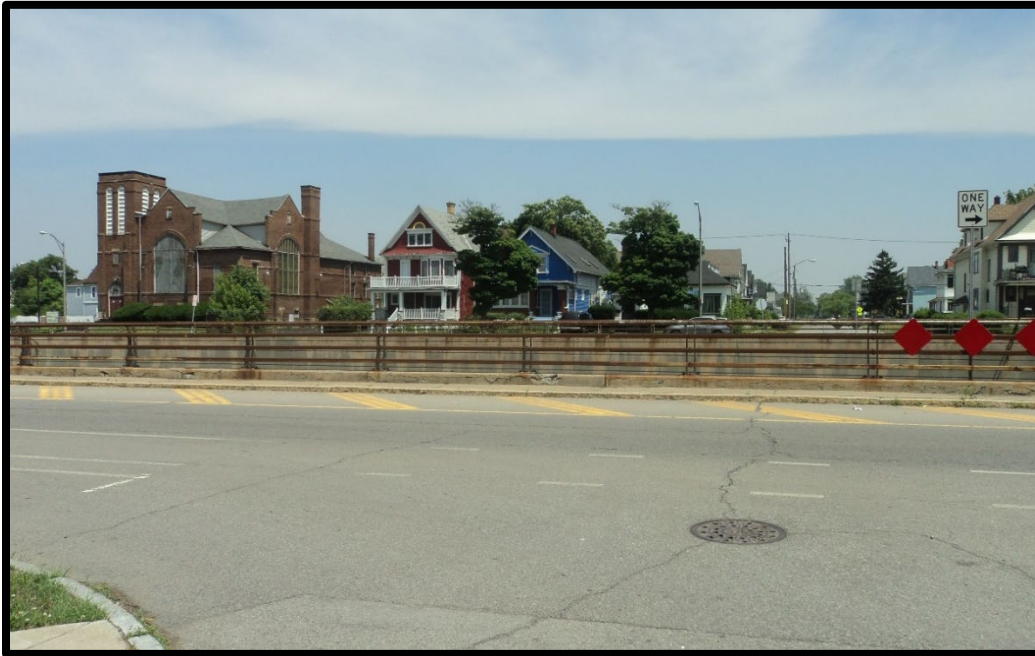
View looking east from Winslow Street and Humboldt Parkway southbound.
