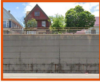
Form-lined Concrete Retaining Wall
